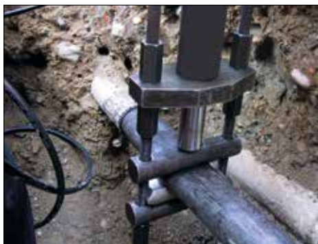
Pumping operation for pipe compressing
