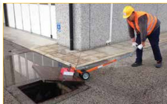
Shownin picture PM500 lifting a steel plate weighing 300 Kg.
