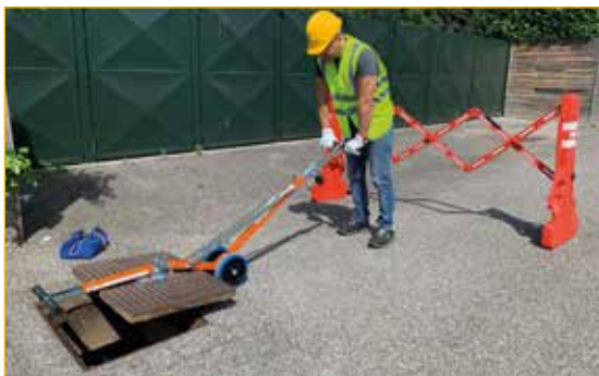
Use 2: opening with wheeled lever APS90 or APS80.
