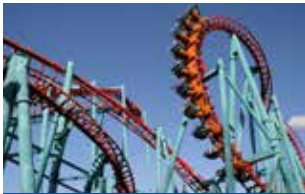
SPECIAL STEEL CONSTRUCTION
